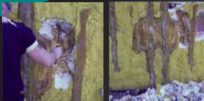
Servicing a Foamed Filled Spa
